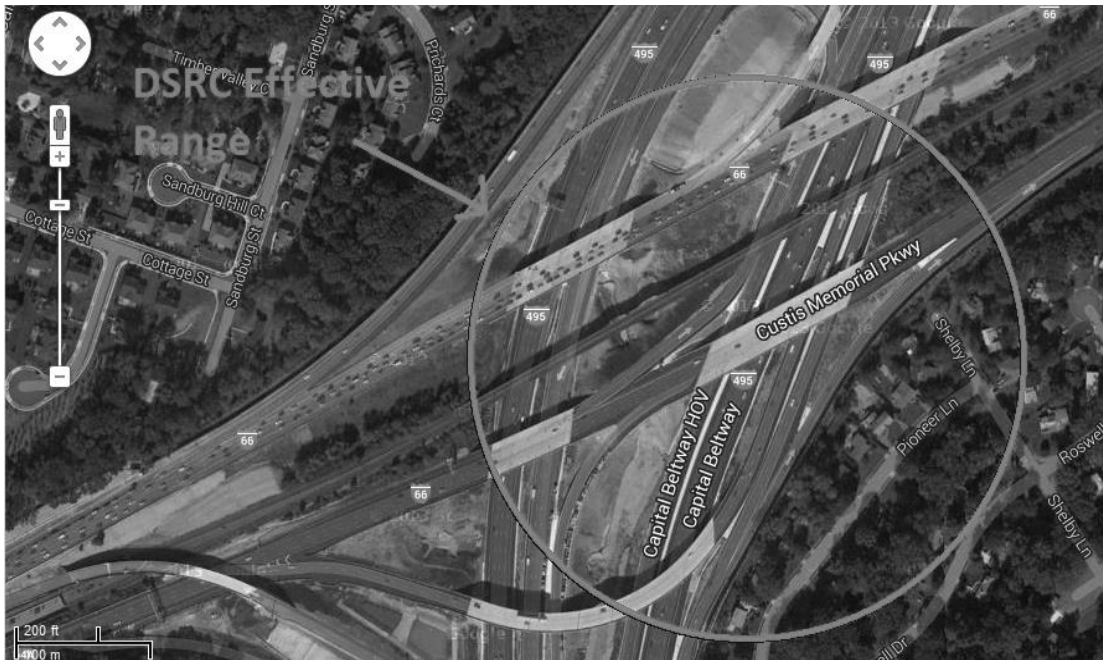
Figure I-3. I-495 and I-66 Interchange Image: Courtesy of CAMP
