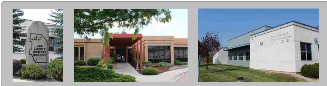
Figure 3-1: Site visit to Boise, Idaho (Source: Noblis 2012)
