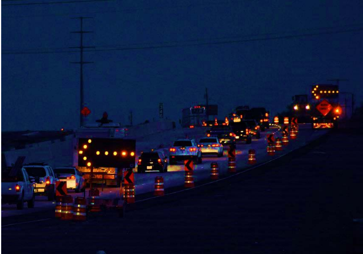
Figure 9. Work Zone with Traffic Control (Source: Texas A&M Transportation Institute)
