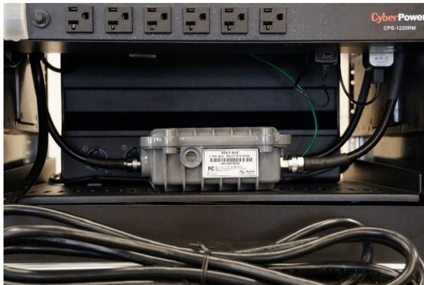
Figure 20. Photo. Mounted RSU.
