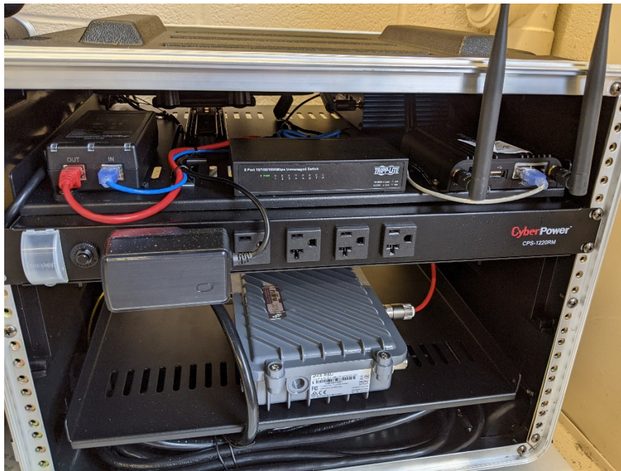
Figure 22. Photo. Power strip mounted below upper shelf.
